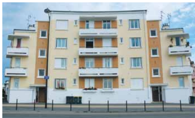
Immeuble 57, rond-point Guynemer (service patrimoine).
